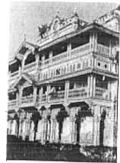
Fig. 12. Street elevation of the Ithnashiri Dispensary.
