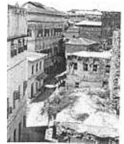
FIG. 20. Characteristic townscape with collapsed buildings.
