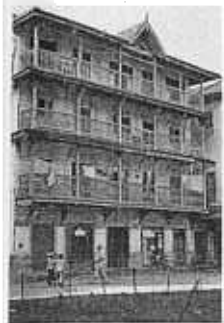
Fig. 11. Street elevation of a building with Indian-influenced stucco work.
